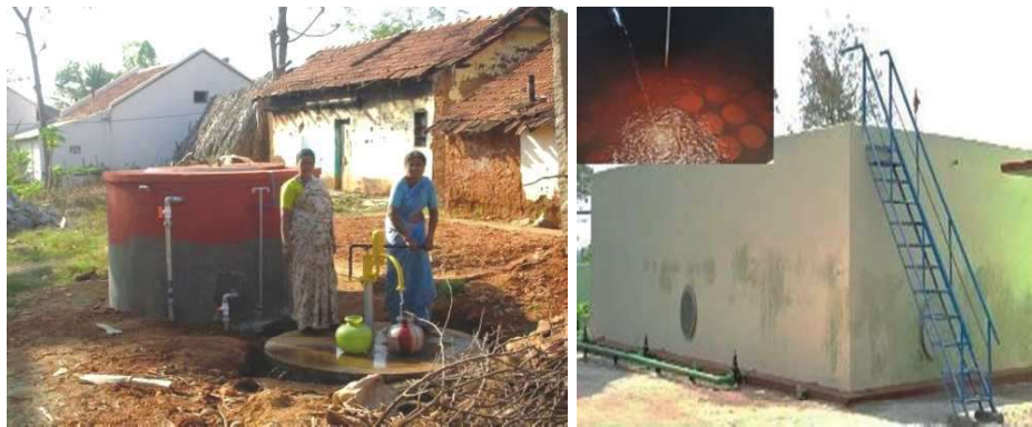
Fig 4. RCC based TERAFIL Filtration unit
