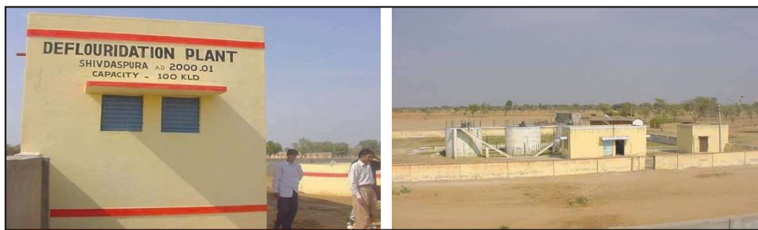
Fill & Draw Defluoridation Demonstration Plants Installed by NEERI Full Scale Plant , 2.27 MLD, Installed at Kadiri (AP)
