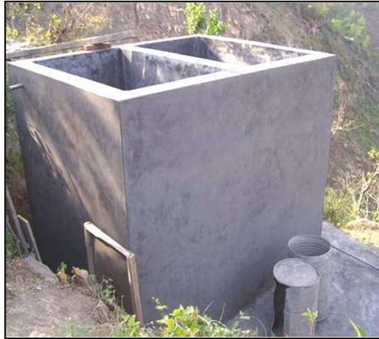
Slow Sand Filtration Unit under construction at village Chhati, Tehri Garhwal, HP
