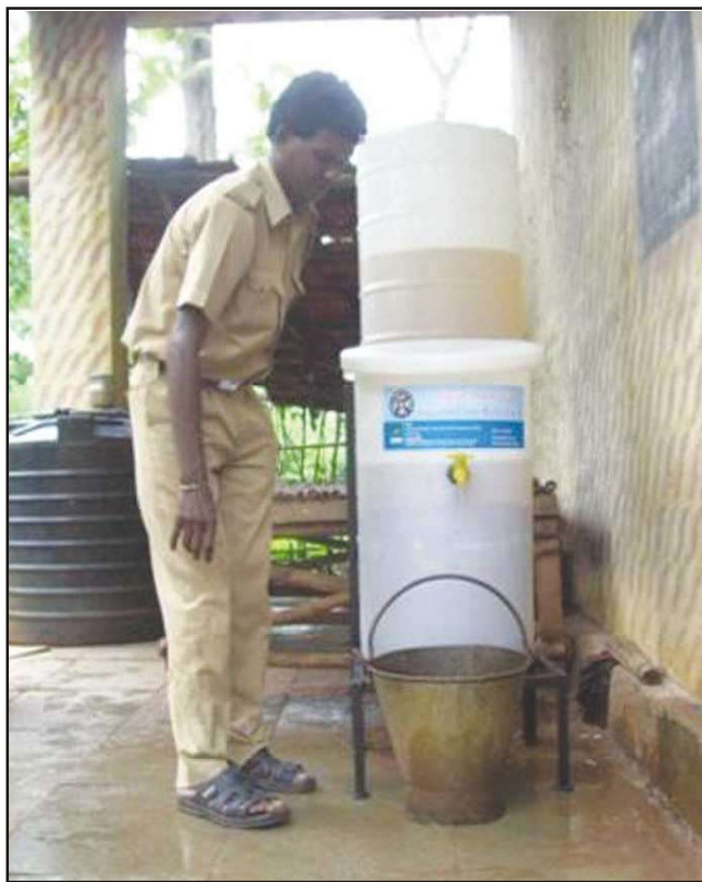
Domestic Iron Removal Units installed in Tadoba Tiger Reserve Forest, Maharashtra for supply of water to Forest Guards
