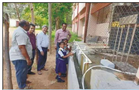
First system installed at industrial biotech park, Jammu
