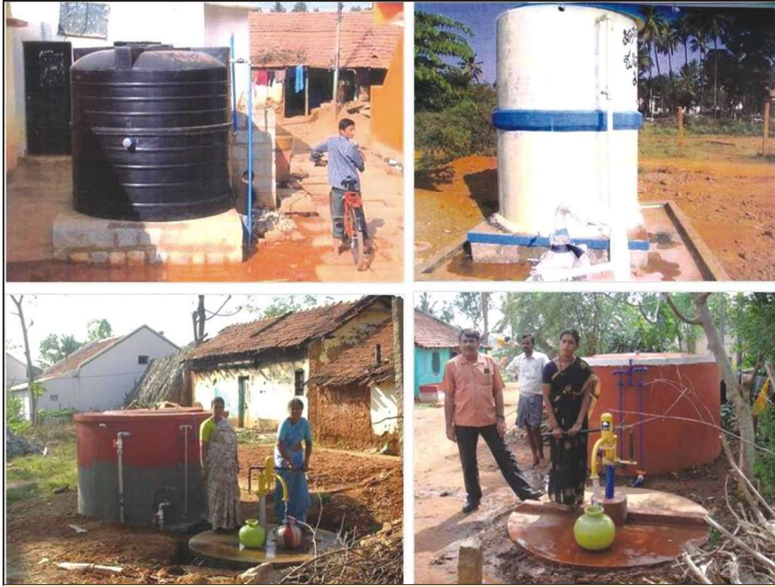
Fig 7. Installation of 5,000 Litre/day Capacity TERAFIL plant in Karnataka by PRED, Govt. of Karnataka
