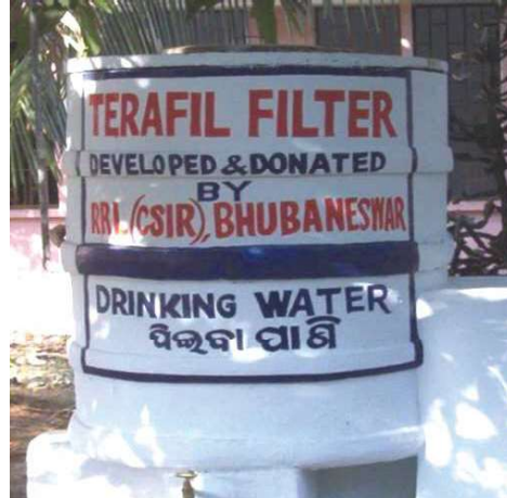
Fig 3. Ferro-cement ring based TERAFIL Filter
