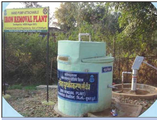
HP attachable Iron Removal Plant FRP Structure (Can be pre-fabricated and installed at the site in a few hours)
