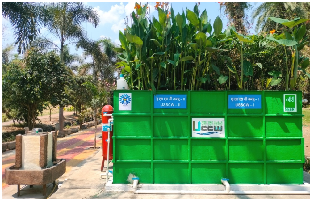
15 KLD UCCW based STP at CSIR – NEERI Nagpur
