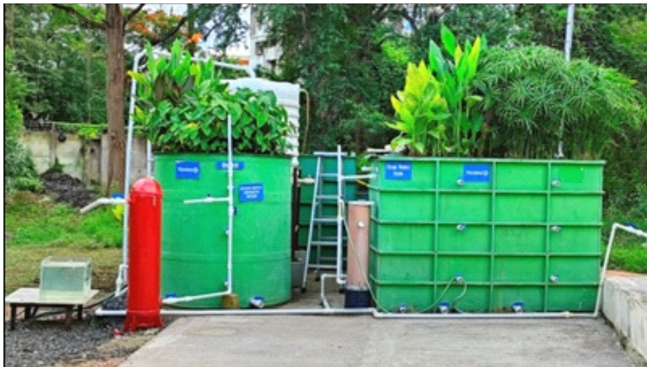
1.5 KLD UCCW based STP at CSIR – NEERI Nagpur
